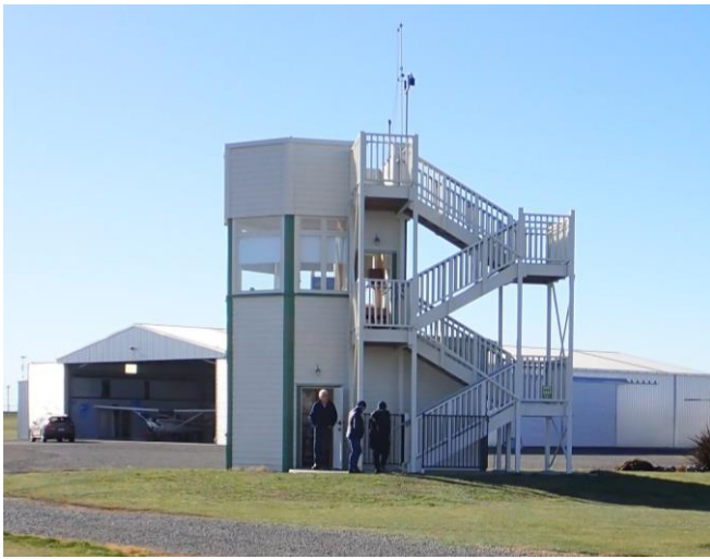
▲ The old Control tower, Warwick Potts, Hillary Milne & Viv Simmons ready to climb up.
